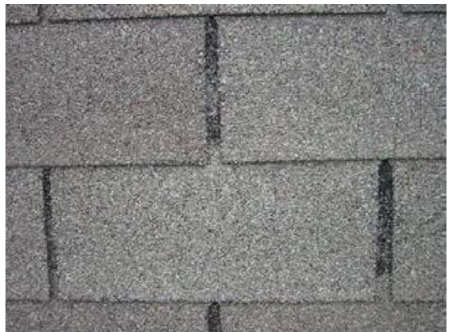
General condition of roof covering.
